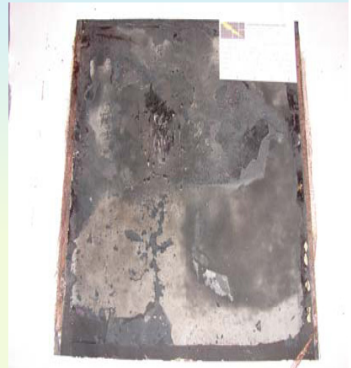
Composite panel damage due to direct lightning strike.
